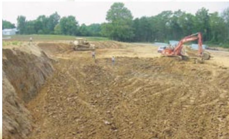
Soon we’ll be pouring concrete for the museum’s foundation!
